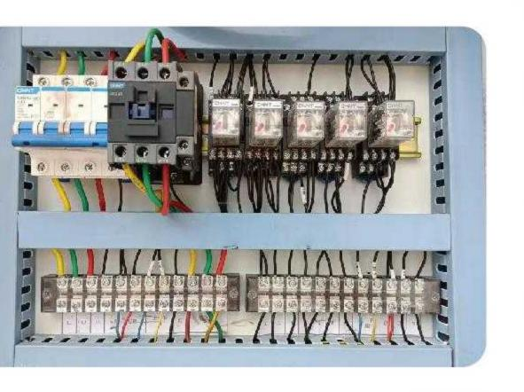
NO.4 独立电控箱 Independent electric control box
